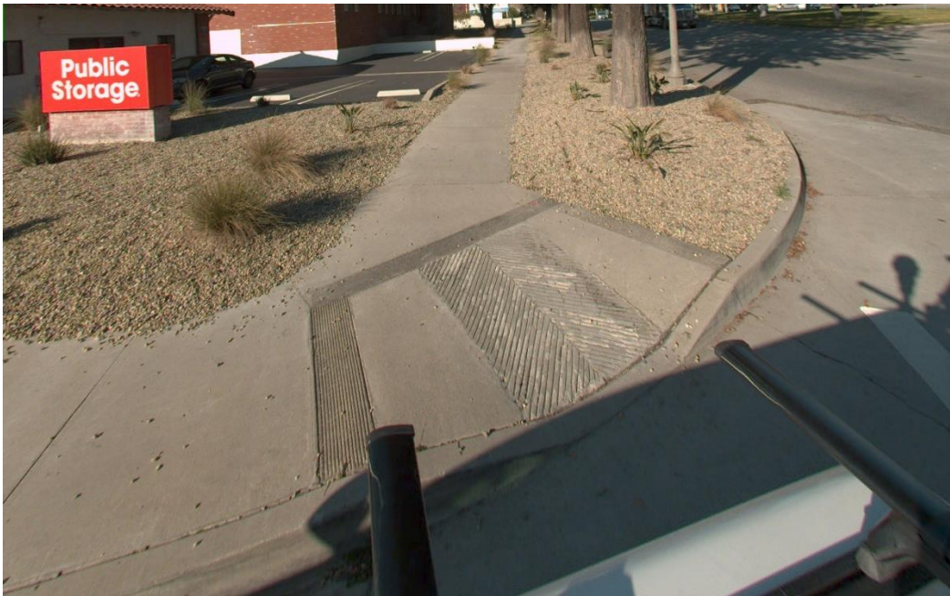
Figure 13 - ADA Conformity Level 3 Ramp
