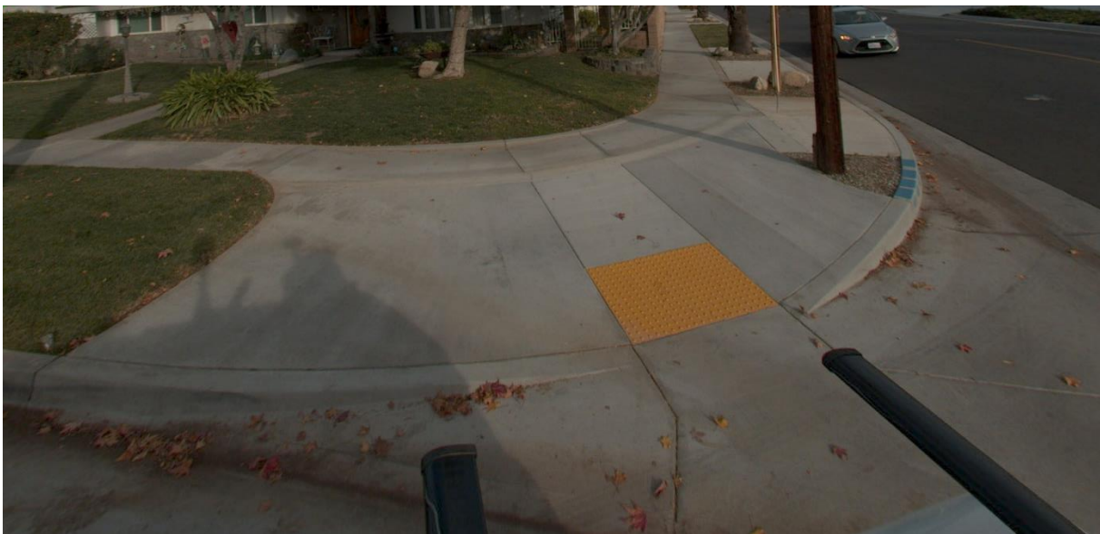
Figure 12 - ADA Conformity Level 2 Ramp
