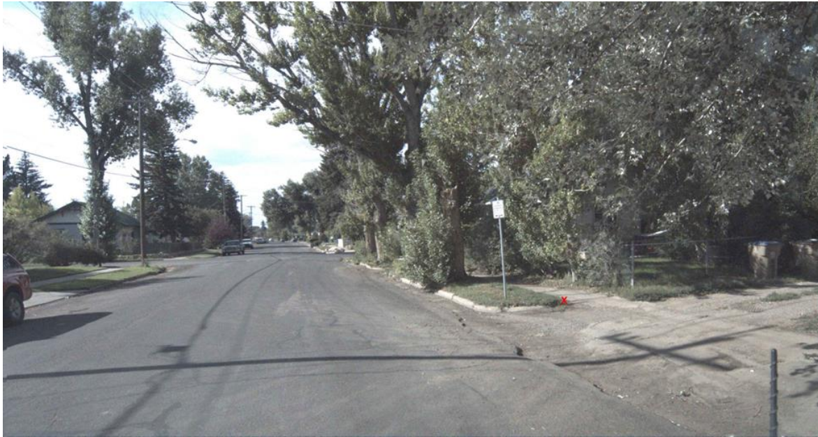
Figure 15 - ADA Conformity Level 5 Ramp
