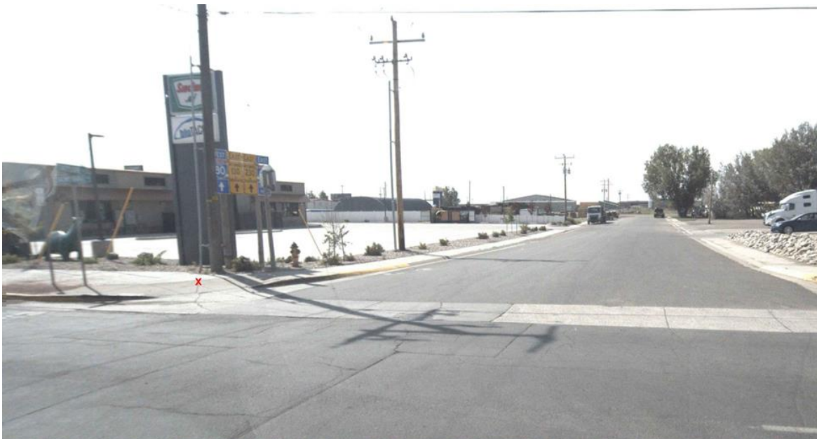
Figure 14- ADA Conformity Level 4 Ramp
